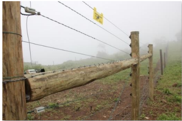
Figure 12. Comprehensive game-proof electric fence with wire mesh at the Aberdare Conservation Area, Kenya.
